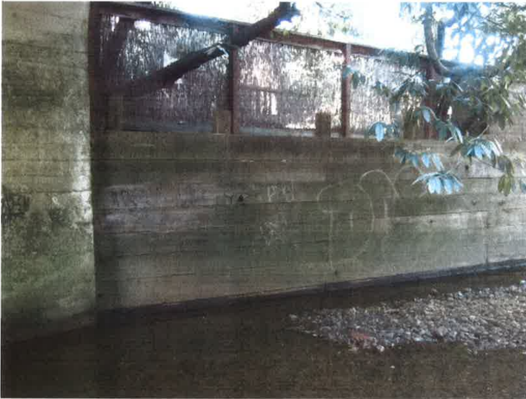
Photo 2. View to Upstream End of Existing Left Bank Retaining Wall Immediately Downstream from the Norwood Avenue Bridge left abutment wall (January 2015).
