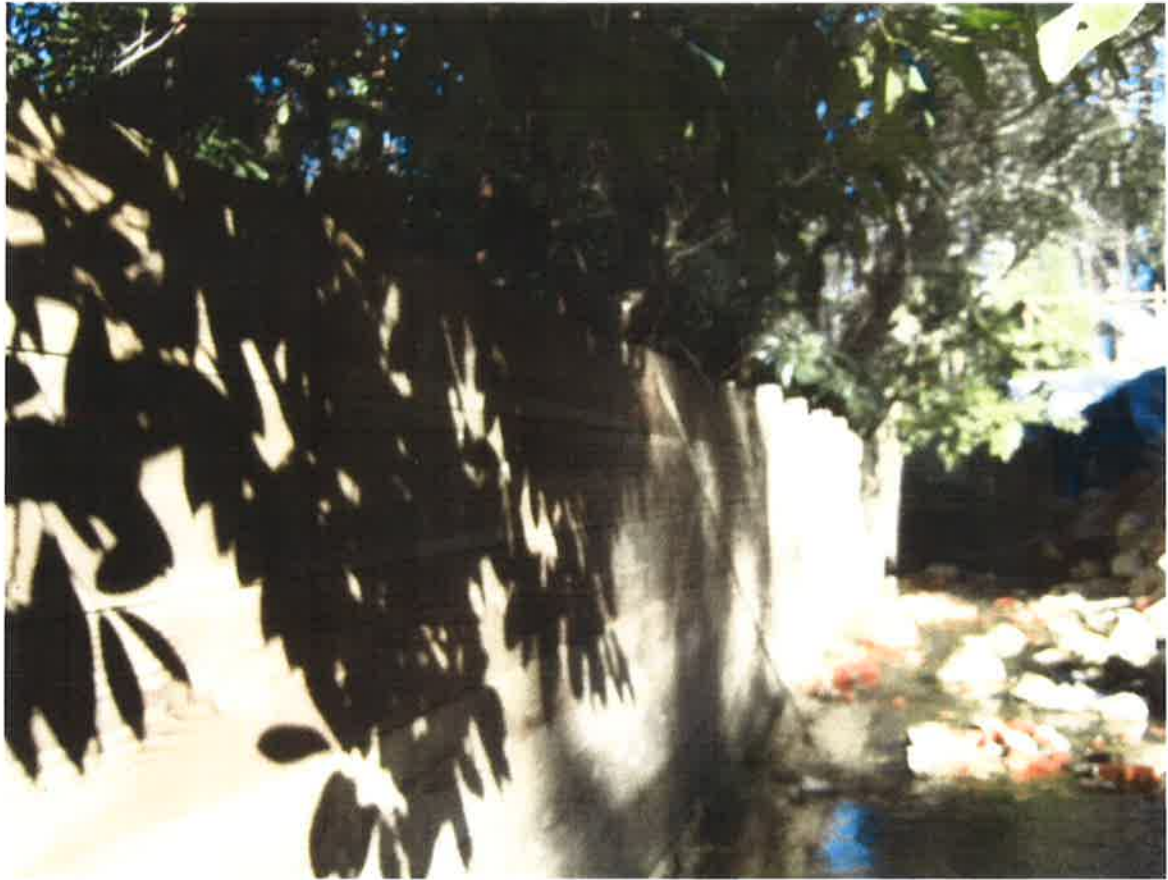
Existing Left Bank Timber Retaining Wall at 14 Norwood Avenue in Ross (January 23, 2015)
