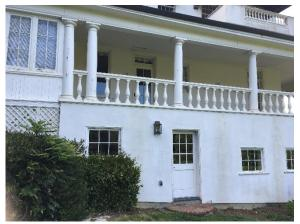
Figure 25: Wrap-around open porch at the main level.
