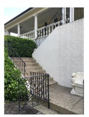
Figure 6: Detail view of double U-shape staircase with concrete steps and metal balustrades.
