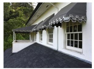
Figure 27: Typical windows with fabric awnings and one of two projecting balconies at the second story of the southeast façade, looking southwest.
