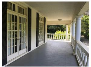
Figure 10: Two sets of paired French doors with transoms and wood shutters north (right) of the primary entrance.
