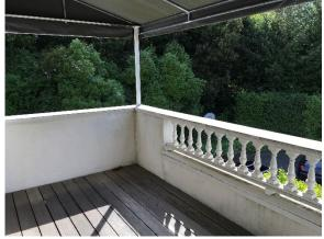
Figure 18: Stucco wall and wood spindle baluster at the second story.
