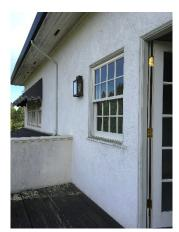
Figure 11: Typical wood eight-over-eight hung window at the second story balcony on the primary façade, looking southeast.
