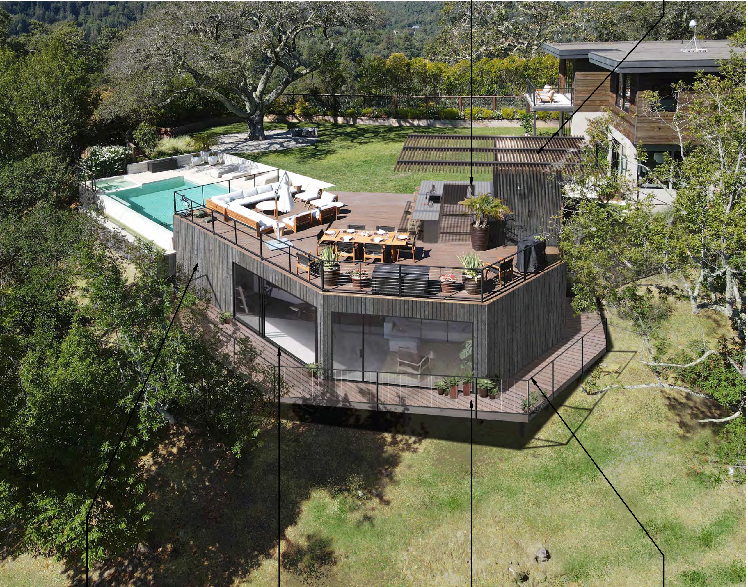
SIDING: WESTERN RED CEDAR RAIN SCREEN WITH SEMI-TRANSPARENT STAIN
