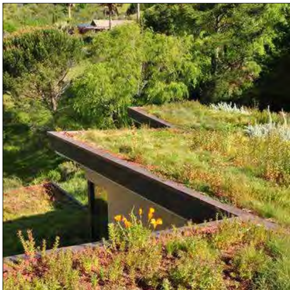
EXTENSIVE GREEN ROOF WITH NATURAL GRASSES
