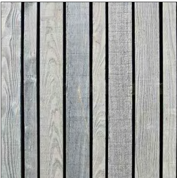
SIDING: WESTERN RED CEDAR RAIN SCREEN WITH SEMI-TRANSPARENT STAIN
