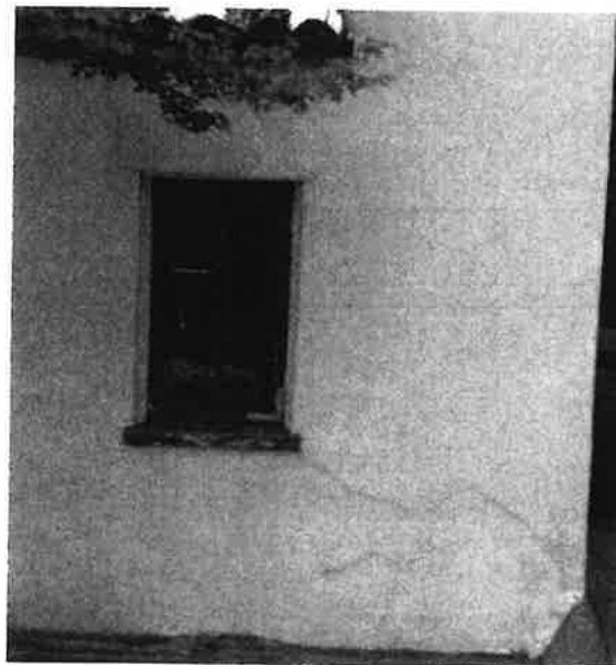
Image 11 and 12: Central firehouse – stucco cracks
