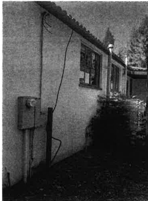
Soil contact with plaster
