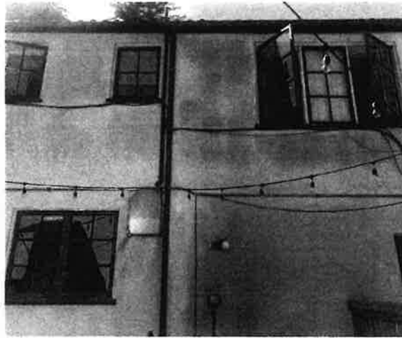
Exposed wiring, faded paint
