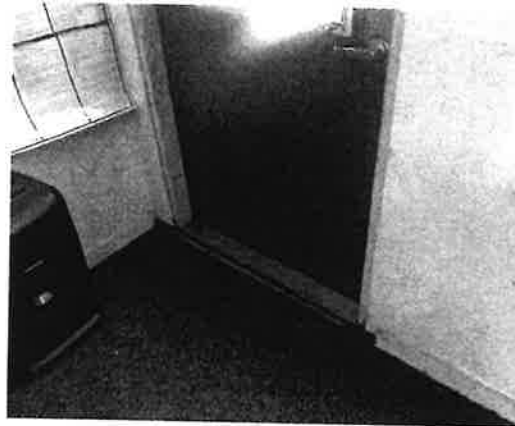
Water staining at threshold
