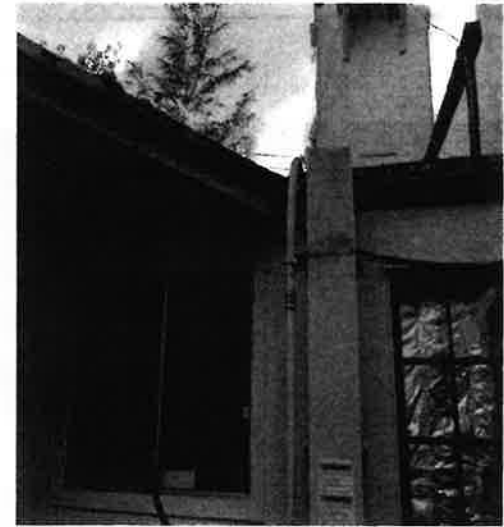
Exposed wiring
