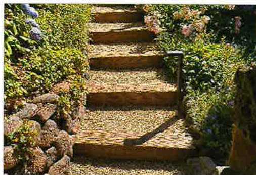
Wood Ties and Crushed Stone
