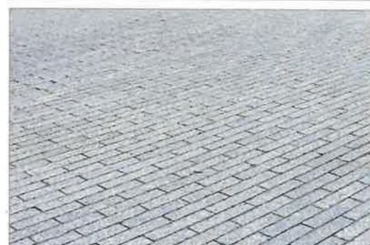
Permeable Concrete Pavers
