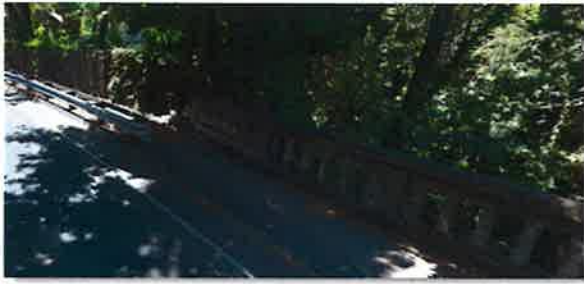
1 Southbound sidewalk gap on SFD Blvd.
