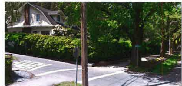
6 Unpaved walkway gaps on Lagunitas Rd.
