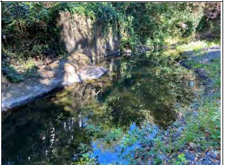
Photo 6. San Anselmo Creek armoring (retaining wall and concrete).
