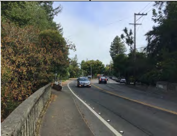
Photo 3. Sir Francis Drake Boulevard Bridge. Facing north.
