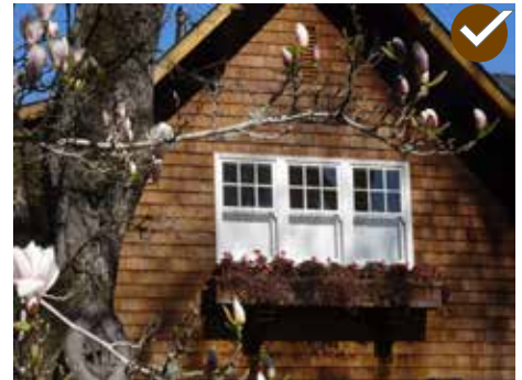
Detailing helps create visual interest and a sense of craftsmanship, while reducing a building's perceived size.
