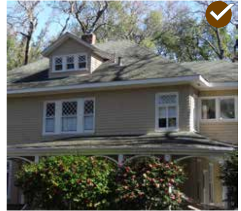
Establish a sense of human scale in the design of a building. The building above incorporates a one-story porch to convey a pedestrian scale.
