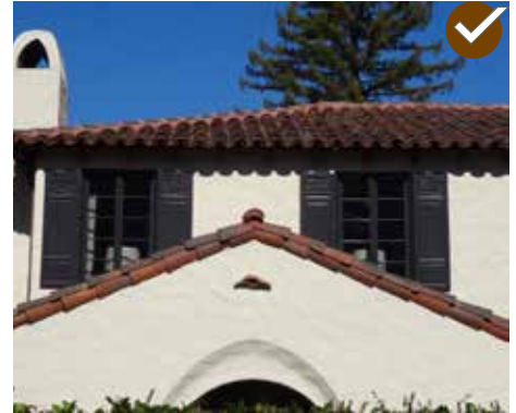
Preserve a significant character-defining feature.
