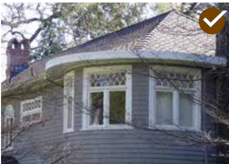
When replacing a window, choose a window that fits within the existing opening and that matches the design of the existing windows on the elevation.
