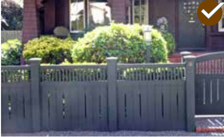
Design fences, walls and landscape buffers to be in scale with the pedestrian.
