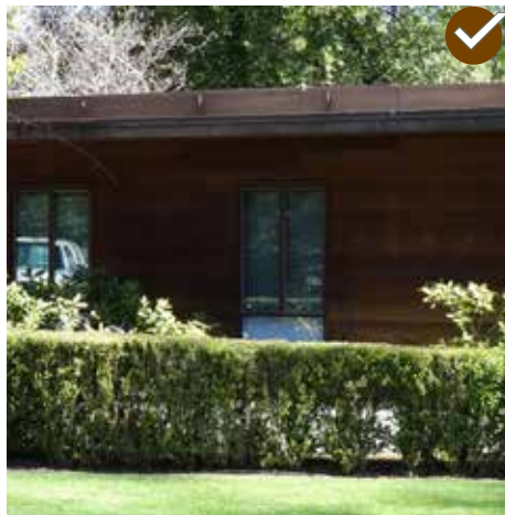
Incorporate low-scale plantings along a street edge to maintain views through to the property.
