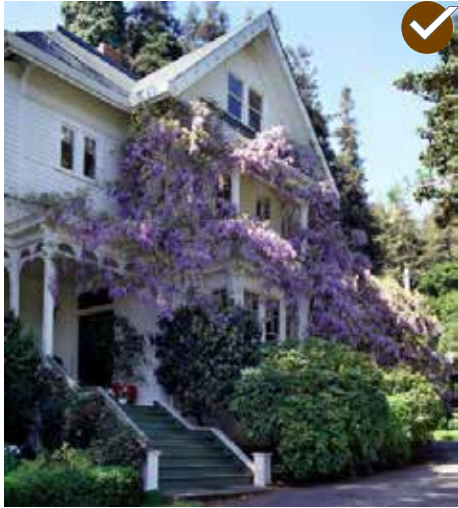
Respect the original design character of the building.
