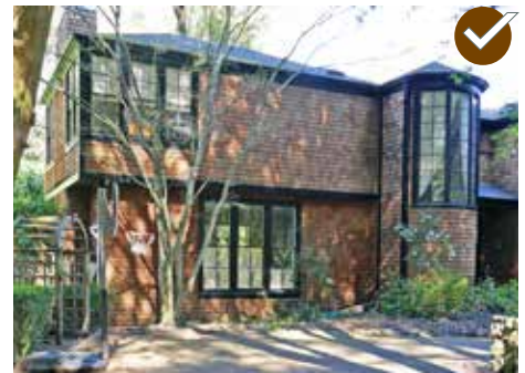
Use vertical and horizontal articulation design techniques to provide a human scale and to create visual interest.
