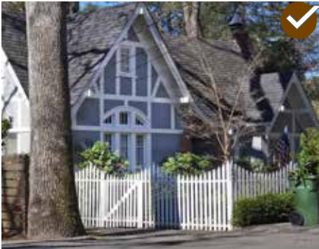
Design a fence or wall to complement the architectural style and character of the building.
