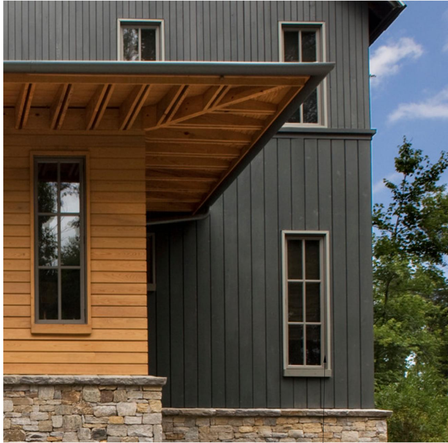
1.5" PROTRUDING CASING DETAIL
