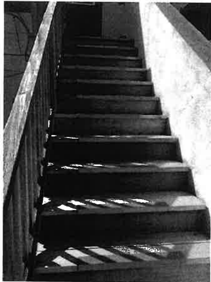
Recently Renovated Treads and Risers
