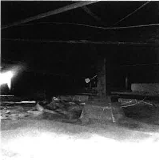
Under floor of Police Station
