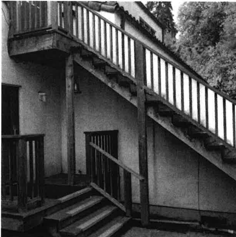
Image 8: Central firehouse dorm access stair (residential construction)
