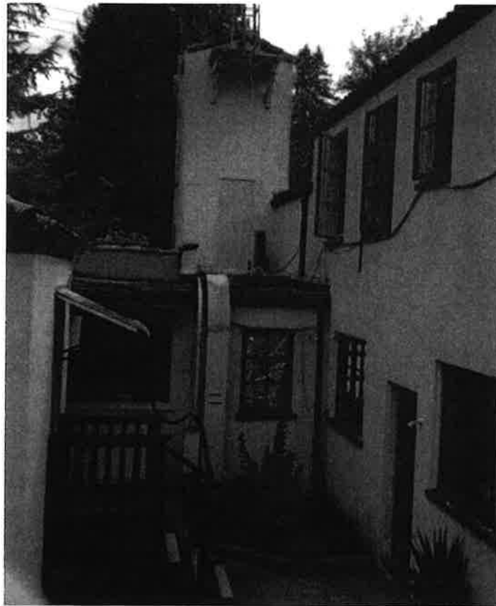
Image 6: Infill between central and north wing
